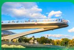
Floating Bridge Moscow
